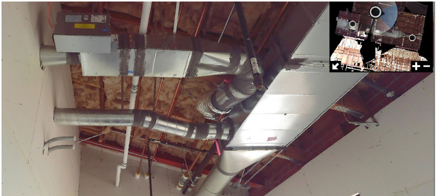
5. As-Built Point Cloud model – Photo realistic view from scanner position
